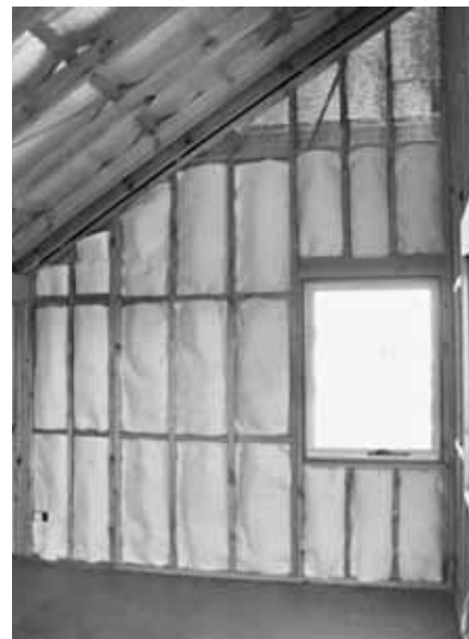
Below: The huge pile waits to be tackled. Right: To maintain an air gap between batts and Air-Cell in the walls, the batts have been stapled to the front edge of the frame.
