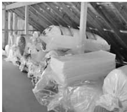
Below: The huge pile waits to be tackled. Right: To maintain an air gap between batts and Air-Cell in the walls, the batts have been stapled to the front edge of the frame.
