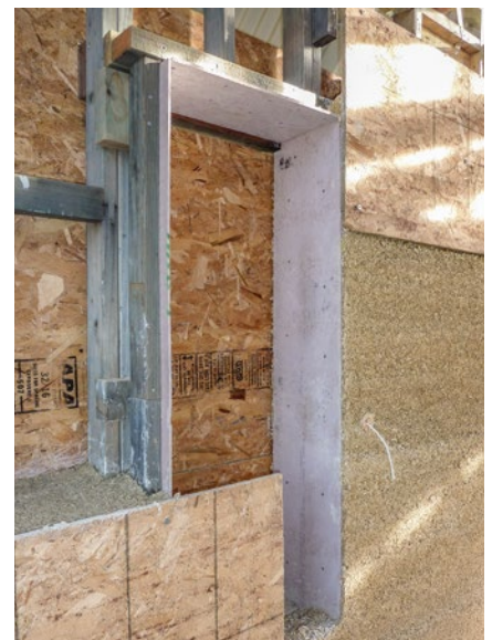
Clockwise from top left: Two-storey gable ends needed some formwork changes. Blocks of wood helped close the gap between formwork and frame. Boxing around openings for a neat finish. Large holes in the ply bracing along with timber wedges helped the hempcrete key properly.
