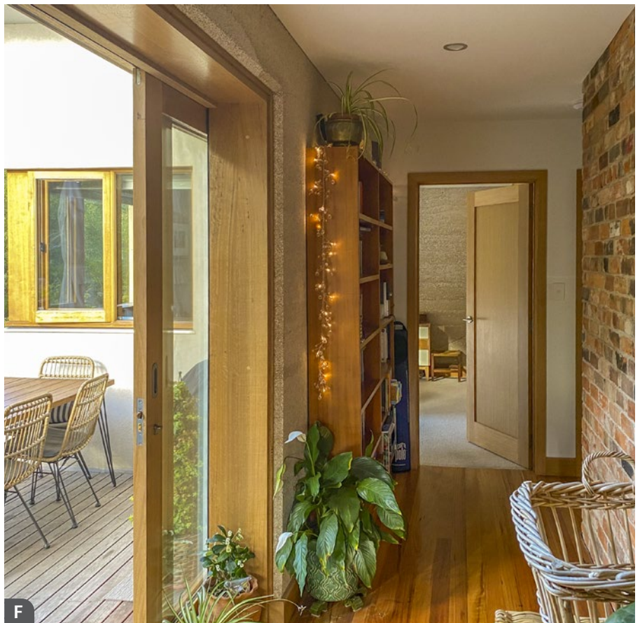
Clockwise from above: The internal recycled 1830s brick thermal mass wall continues up through both floors. Available winter solar gain is maximised through the large double glazed sliding doors, hand made from Tasmanian oak by Andrew Otto. Floors are silvertop ash.
