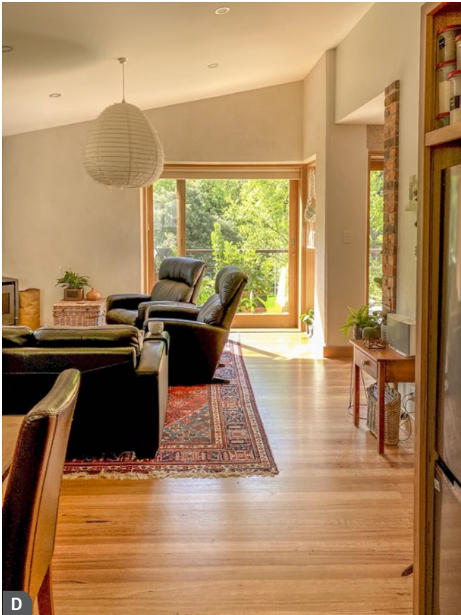
Clockwise from above: The internal recycled 1830s brick thermal mass wall continues up through both floors. Available winter solar gain is maximised through the large double glazed sliding doors, hand made from Tasmanian oak by Andrew Otto. Floors are silvertop ash.
